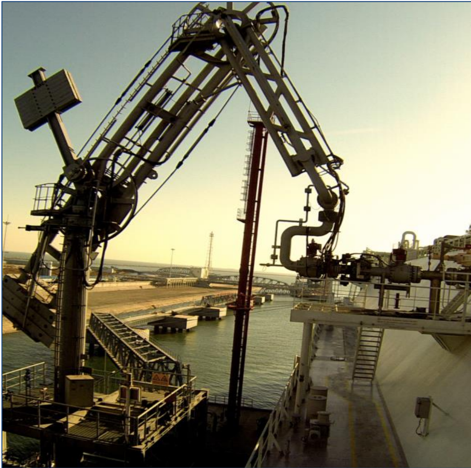
Image 31 Firefighting tower and HP gas export pipeline – HP gas export manifolds
